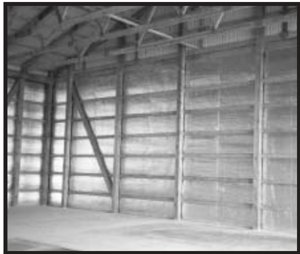
Foil insulation installed with a finishing ceiling
